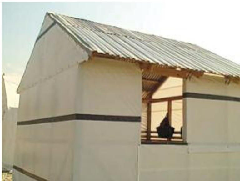
Top: Bodies of quake victims are still buried in this unstable building. Above: The Red Cross hastily erected such shelters.
